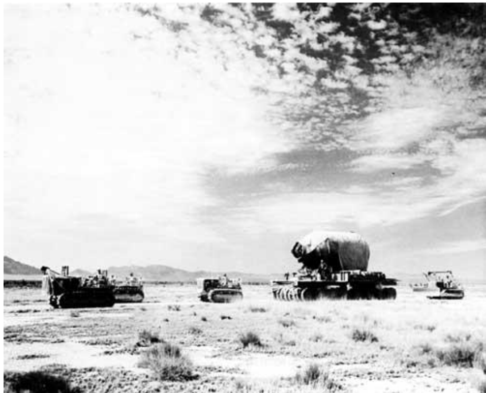
Figure 39. Jumbo moving to Trinity Test Site (1945). ( Courtesy Los Alamos Photographic Laboratory )
