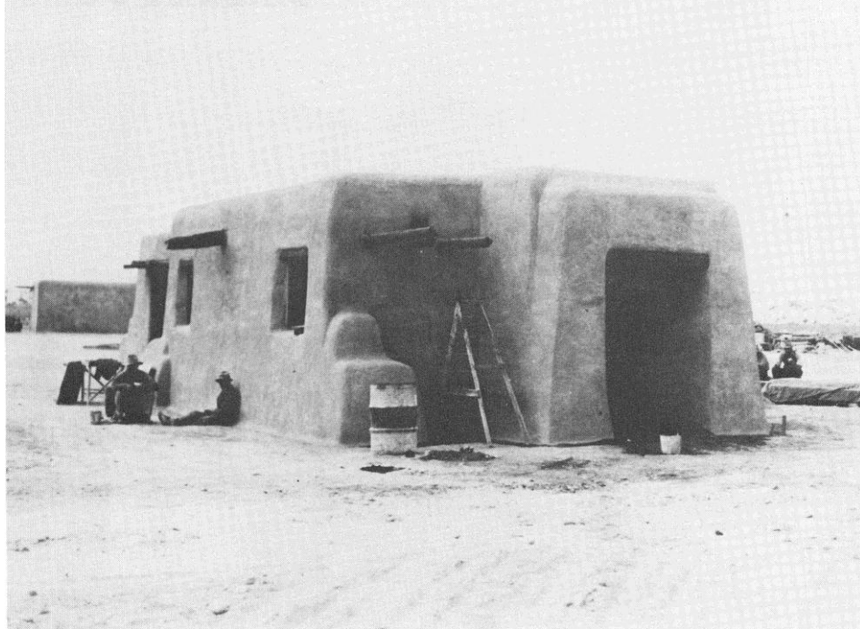
Figure 15. Adobe style of construction by New Deal Agency Work Crews (1930s). (Courtesy White Sands National Monument)
