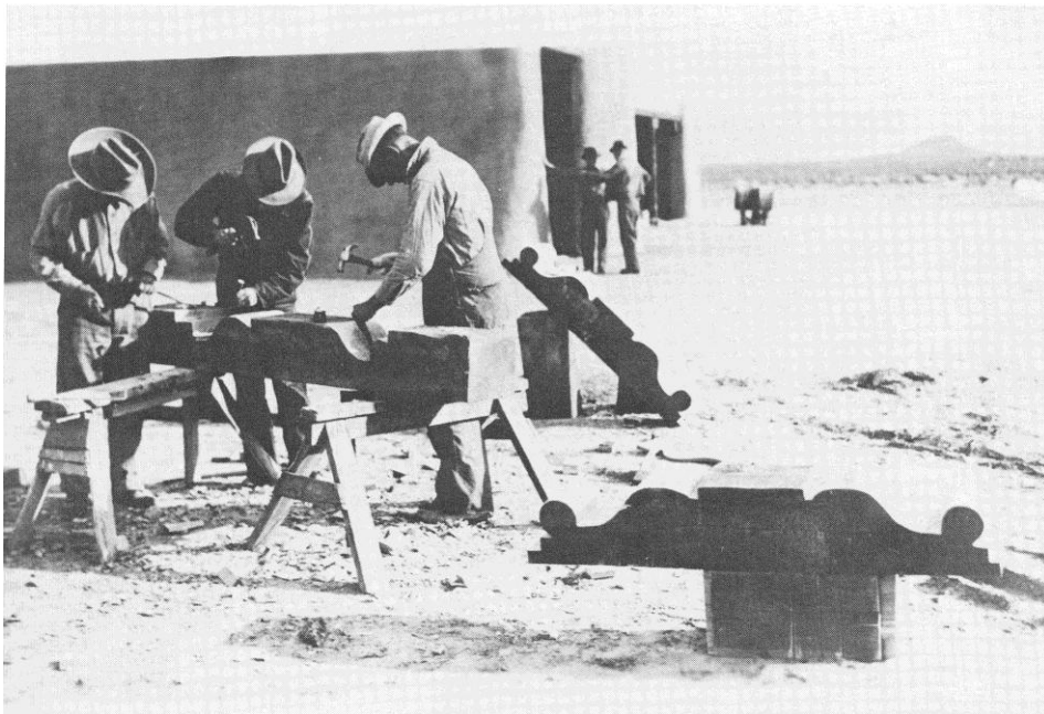
Figure 16. Hispanic woodcarvers making corbels for Visitor Center (1930s). (Courtesy White Sands National Monument)
