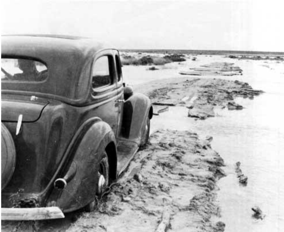
Figure 33. Clay-plated road washed out by heavy rains (1940s). (Courtesy White Sands National Monument)
