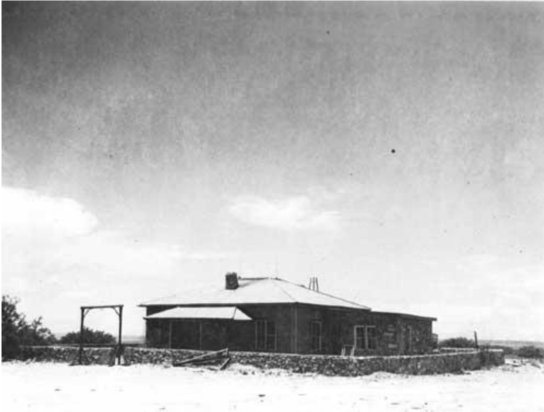
Figure 37. McDonald Ranch (1945). ( Courtesy Los Alamos Photographic Laboratory )
