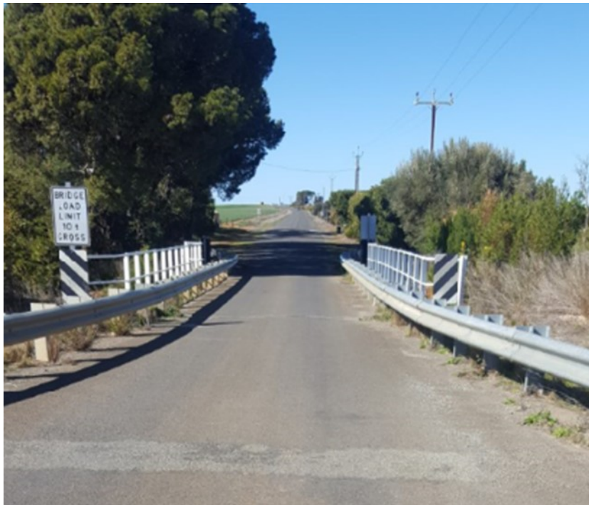
Hampden Bridge with 10 ton mass limit in place
