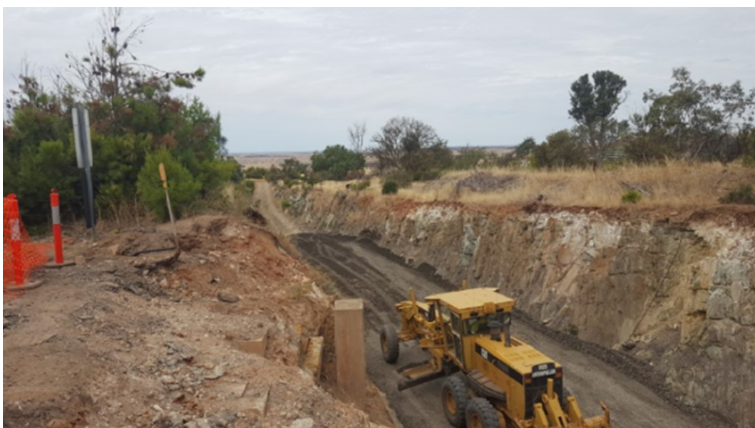
Works infilling the rail corridor
