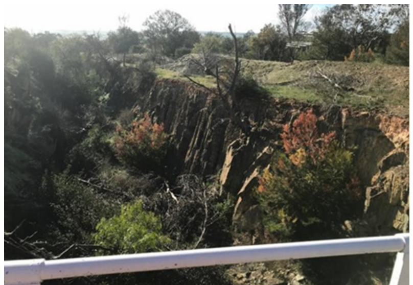
Northern bridge support, corridor prior to works
