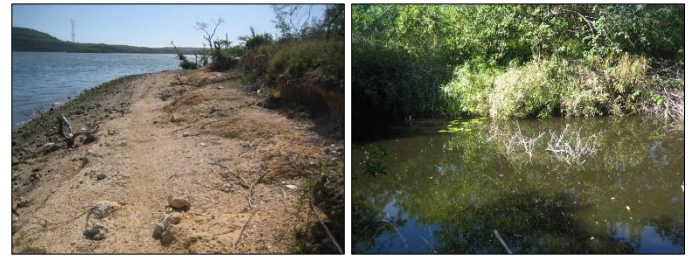
Fig. 5. Threats include erosion of the seashore (left) and impacts of invasive plants and river bank erosion along El Cobre River (right).
