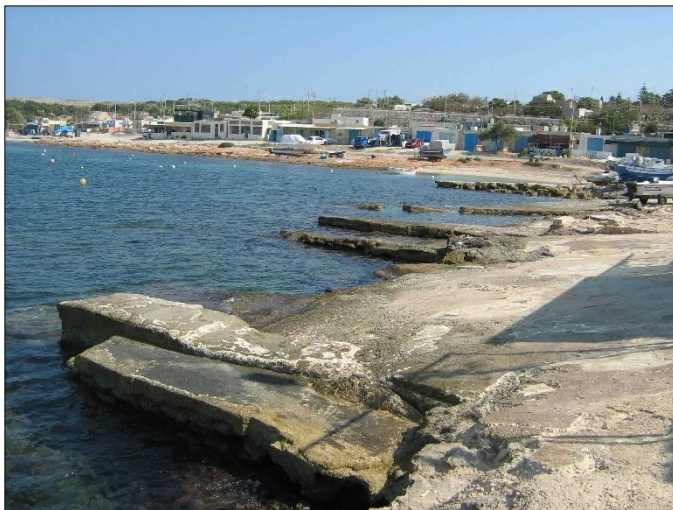
Fig. 1. Jetty structures at White Tower Bay; a highly modified shoreline.
