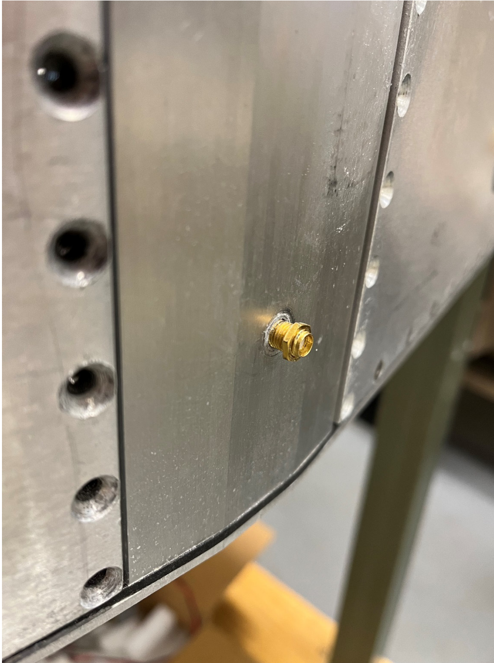
Figure 4. Photo of corrosion following the unscrewing of the nut on the SMA connector
