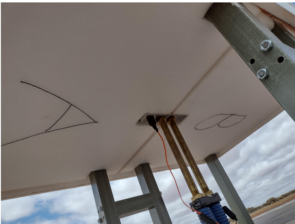
Figure 9: The foam covers on the underside of the antenna.
