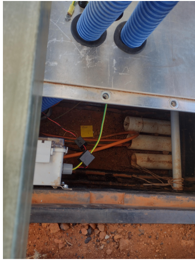
(a) The ferrites on the DC power lines in the pit. (b) The ferrites at the DC input to the antenna.
