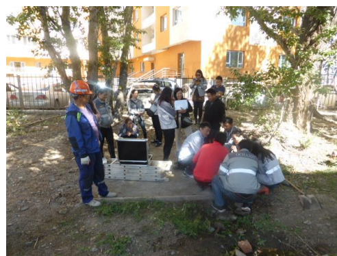
On-site training in installation of mechanical equipment in Ulaanbaatar
