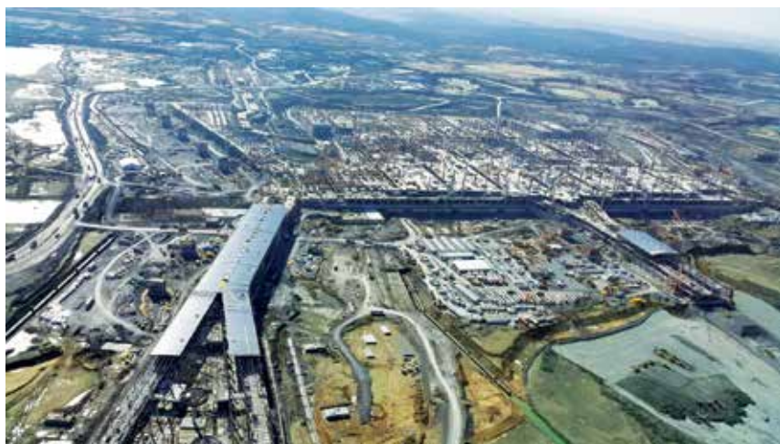
Construction of the Third Istanbul Airport.
