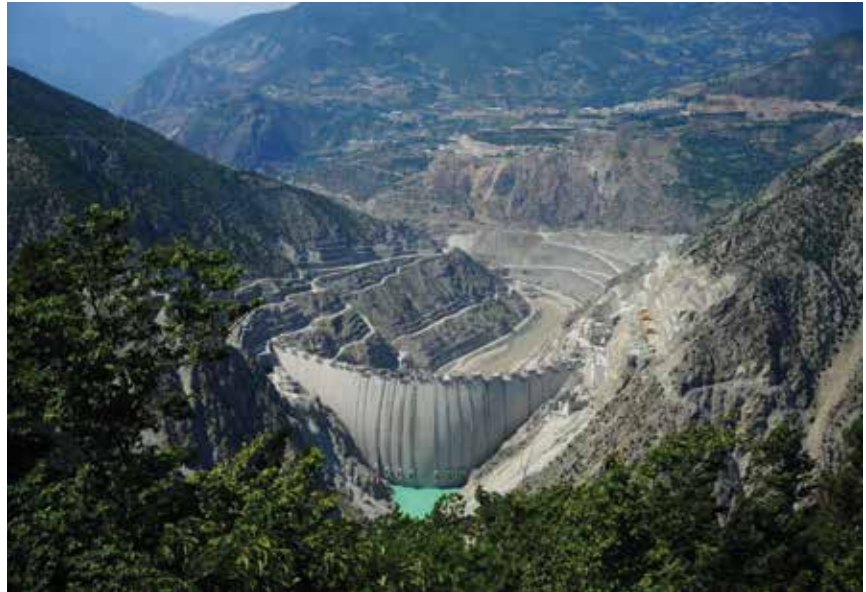
HPP construction in the Black Sea Region. Source: ekopangea.com
