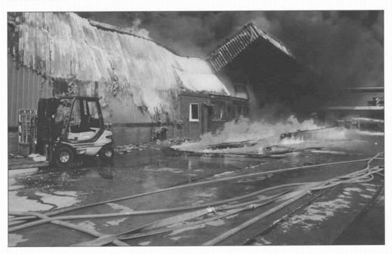
*Figure 4:* The loading bay side of the raw materials warehouse with collapsed walls and canopy, and molten flaming chemicals flowing down the ramp. Courtesy of West Yorkshire Fire Service.
