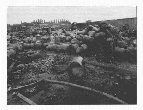
*Figure 14:* Drum storage areas at X and J-Bays looking towards finished goods warehouse. Contaminated water can be seen flowing from the area.
