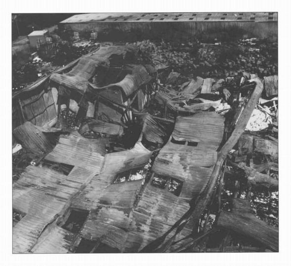
*Figure 6:* The burnt out raw materials warehouse showing collapsed roof, and remains of the oxystores at the top left of the building. The scorched finished goods warehouse lies behind the open drum storage areas (X and J-Bays).
