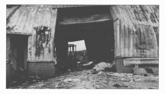
Figure 7: Burnt out entrance to raw materials warehouse with solidified chemicals from storage inside. The door of the office where the records were kept is to the right.
