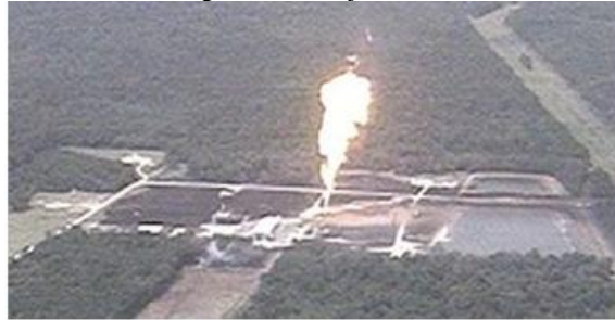
Figure 7 Fire after complete rupture of the well head in Moss Bluff 20 August 2004
