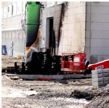
Figure 5 Burnt wooden pallets after the Ghislenghien accident (130 m from rupture)
