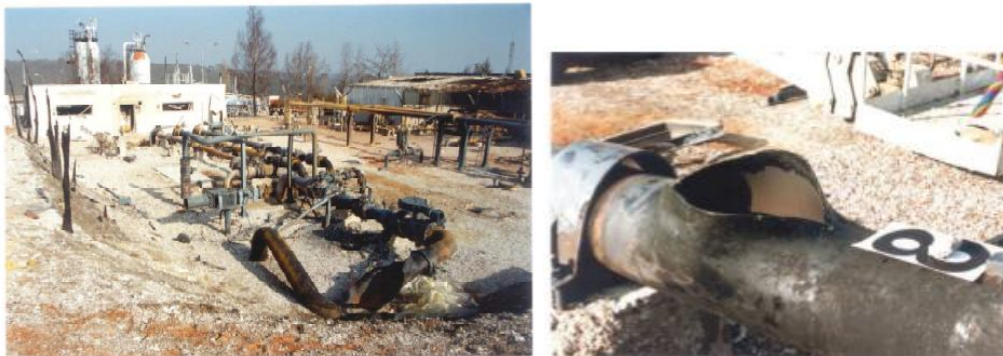
Figure 3 Image of ruptured pipes after the Saint-Illiers accident in 1996
