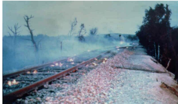
Figure 1 Nearby railroad after Velaux accident in 1977
