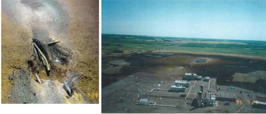
Figure 4 Image of the pipe and damages around the crater after the Rapid City accident in 1995
