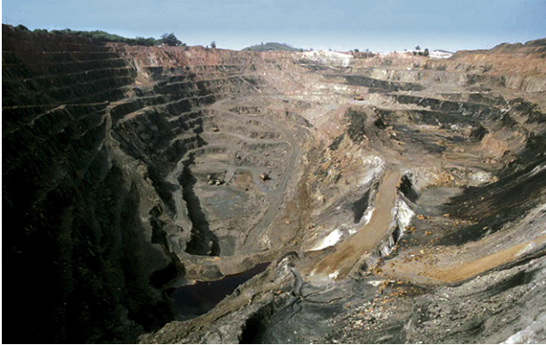
Figure 11. Tharsis mines. Aspect of the open pit from Northern Vein before being closed and flooded.
