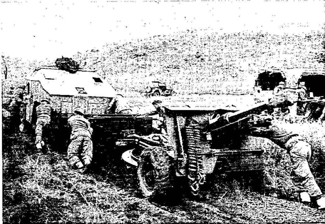
Movement on deeply rutted tracks.
