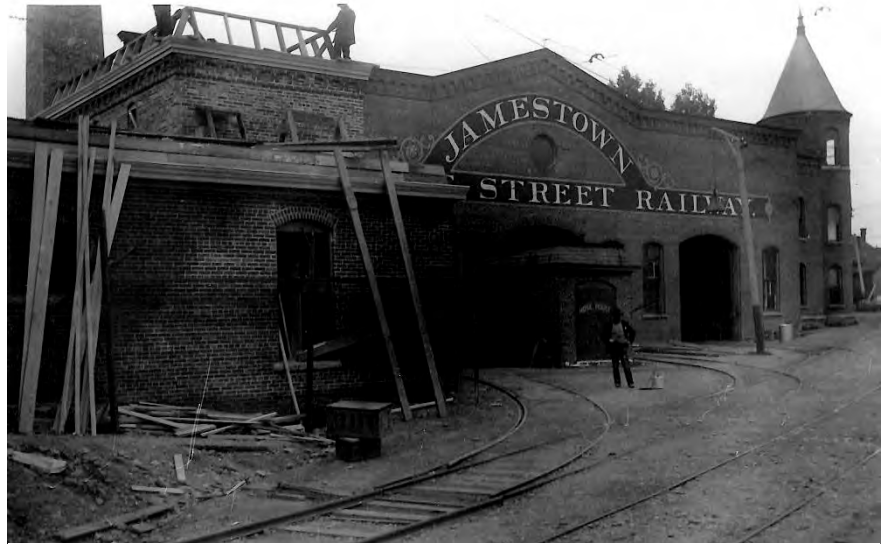
The Street Railway Car Barn under partial construction
