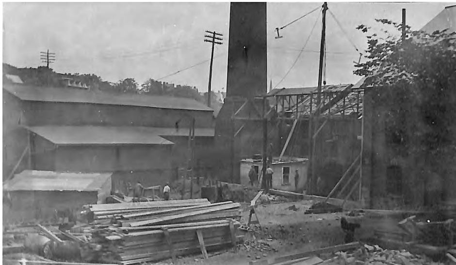
Broadhead Power House under construction
