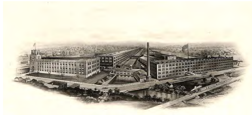
Wide angle view of the entire Dahlstrom complex
