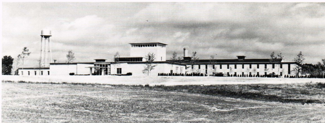
Fig. 12—Building 1 at Howard County, the first University-owned home of APL, dedicated October 16, 1954.
