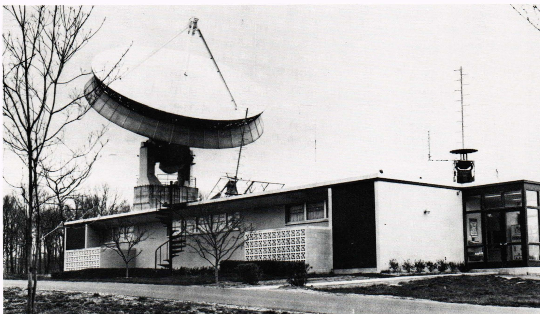
Fig. 16 —The Injection Station epitomizes the Transit program. Through the 60-foot-diameter radio telescope, a special computer supplies data to the memory of the satellite. The same telescope is used to track satellites and receive signals of scientific interest from the sun and other regions of space.
