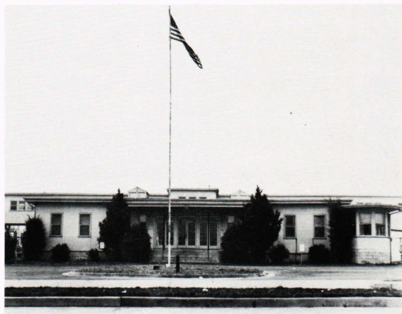
Fig. 6—The Main Building at the Forest Grove Station, 9000 Georgia Avenue, Silver Spring, associated with major engineering activities in the Bumblebee Program including telemetry, supersonic aerodynamics, environmental tests, fabrication of the sectionalized Terrier, and location of central machine and electronic shops. Occupied in 1945, it was relinquished in 1962.
