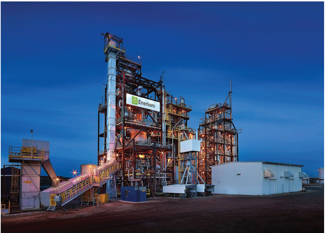
Energkem's biofuels plant in Alberta, Canada.
