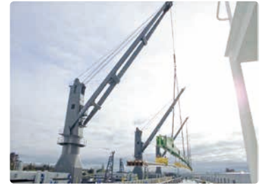
Synchronized Crane (50tons × 3)
