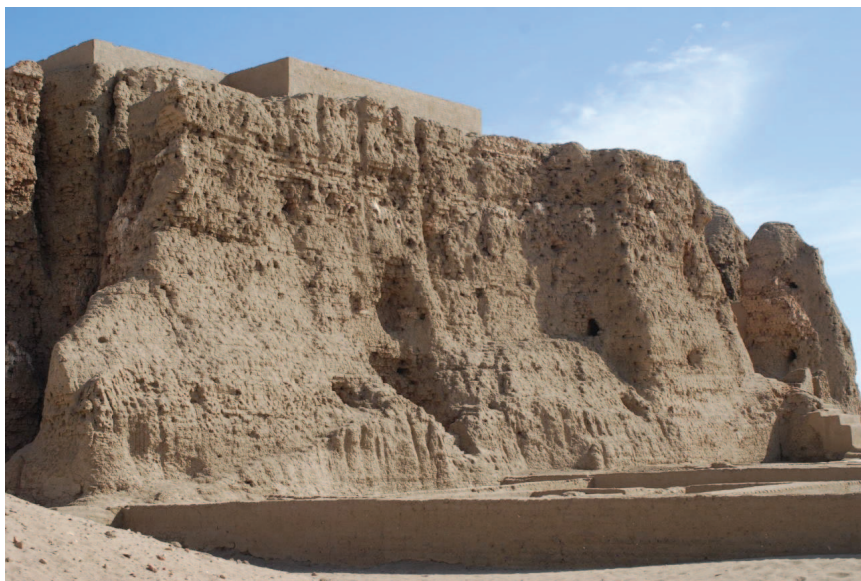
Figure 1. The massive body of the Deffufa (‘mud-brick building’ in Nubian) of Kerma, Nubia. It was built entirely of sun-dried bricks and was the reference structure of the classic Kush civilization (2000–1500 BC).
