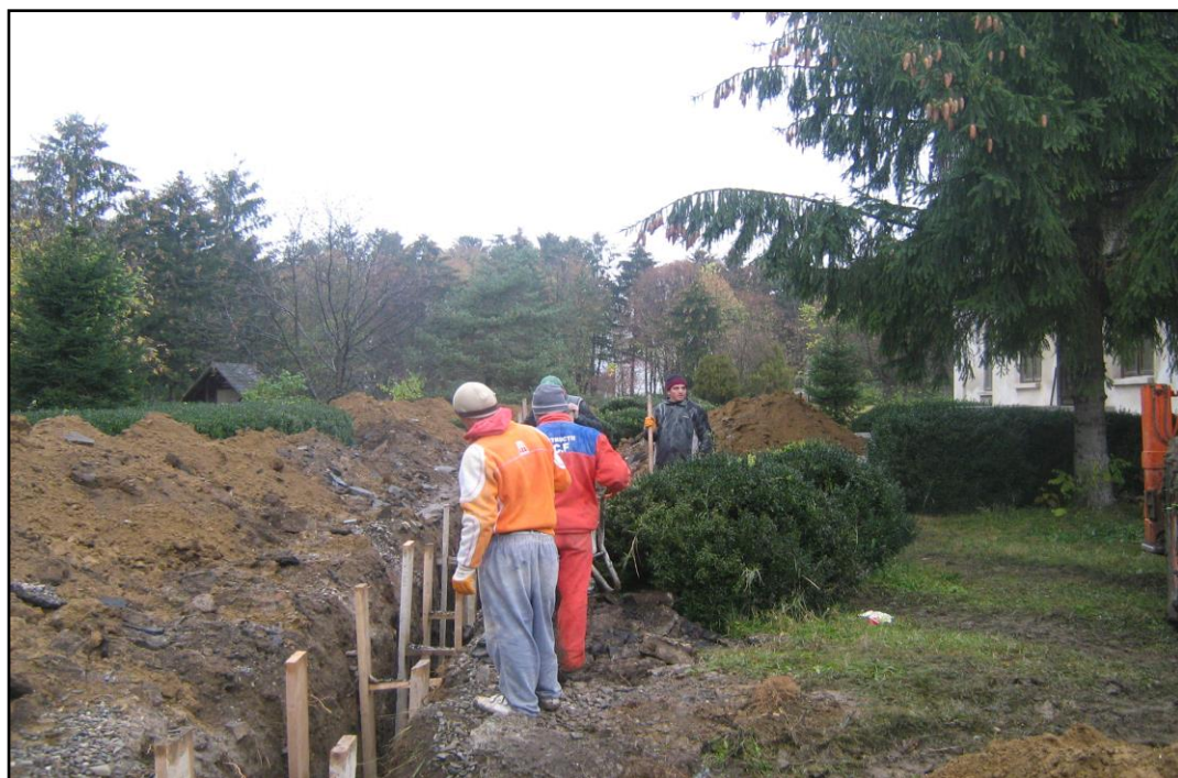
Executare dren perimetral
