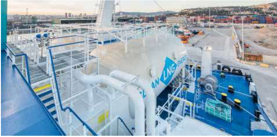
The two Wärtsilä LNGPac on-deck tanks.
