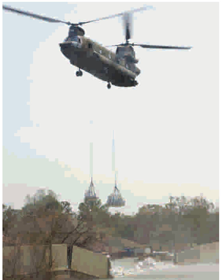
A CH-47 moves into position to drop a sling-load at the break in the 17th Street Canal, 10 September 2005. The 149th Aviation Support Battalion, Texas Army National Guard airlifted and strategically dropped bundles of rock and sand at the break in the 17th Street Canal, which collapsed when Hurricane Katrina hit New Orleans, Louisiana. U.S. Air Force photo by Master Sgt. Scott Reed.
