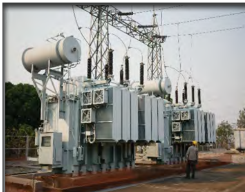
Figure 8-4. Substation showing transformer appropriate for connection to subtransmission (left); detailed diagram of transformer (right)
