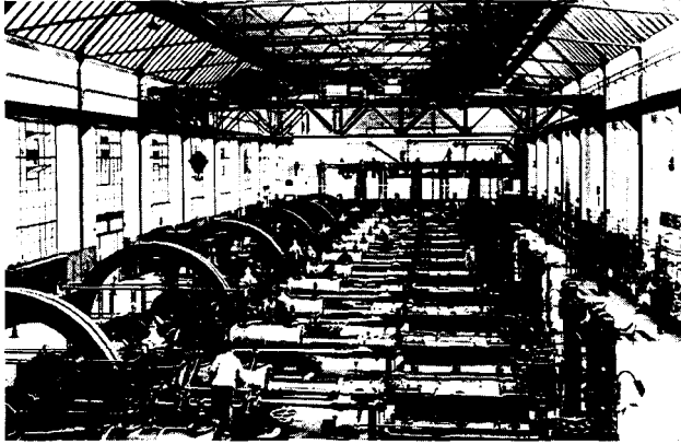
Fig. 55. High pressure lye pumps for gas purification.
