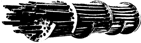
Fig. 7. Destroyed tube cluster from a heat exchanger, 1910.
