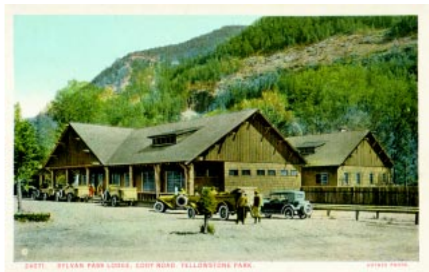
Sylvan Park Lodge on Cody road. 1924.
