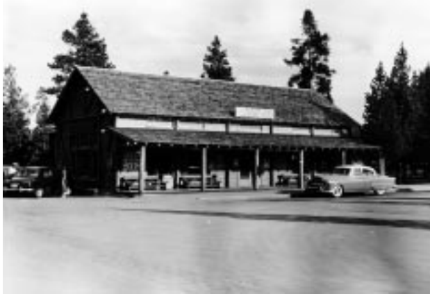
Haynes Photo Shop. 1951.
