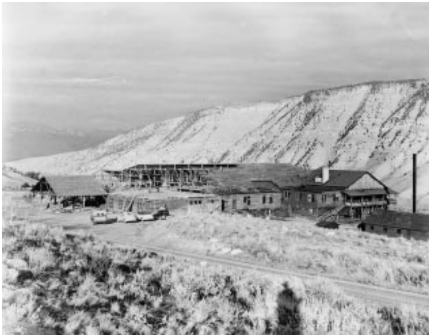
Mammoth Lodge being demolished. 1949.
