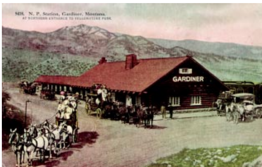
Northern Pacific Station, Gardiner, Montana, at Northern Entrance to Yellowstone. ca. 1910.
