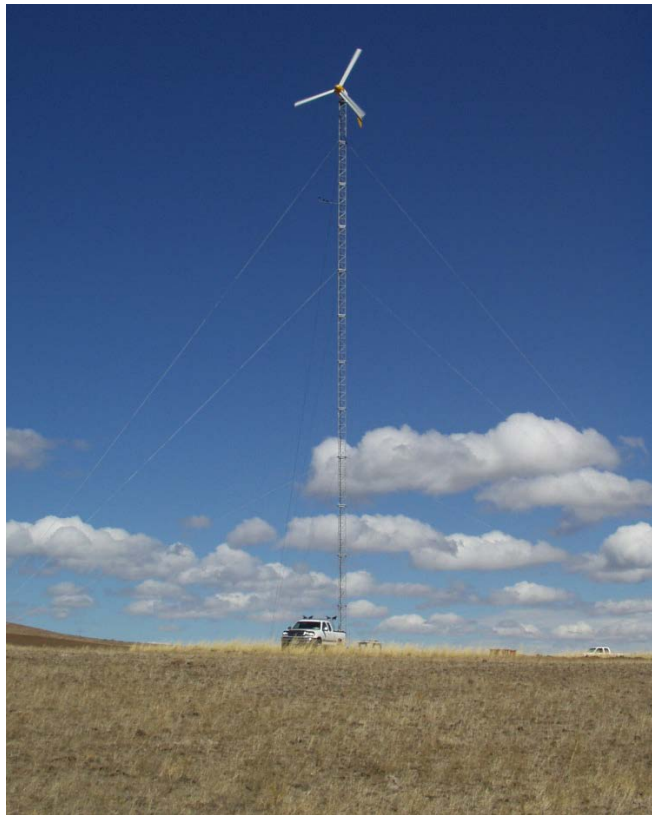
Figure B-1. Bassetti turbine in Klickitat County. Photo by Gwen Bassetti, NREL 26429
