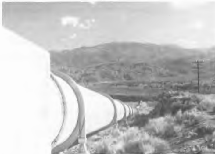
Pipeline that carries water diverted from the Owens River in eastern California to Los Angeles. Because water diversions constructed since the turn of the century have dried up the Owens River, hydropower plants were recently proposed for many of its tributary streams in the Sierra Nevada Mountains.
