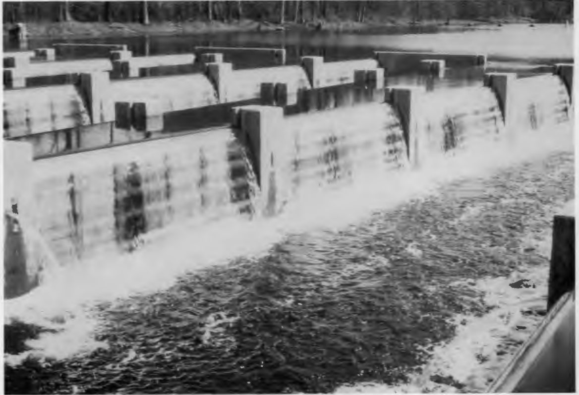
Reregulation weir constructed by the Tennessee Valley Authority below the South Holston Dam. The structure both aerates water discharged from the dam and dampens flow fluctuations resulting from intermittent releases. Photograph by Glenn Cada
