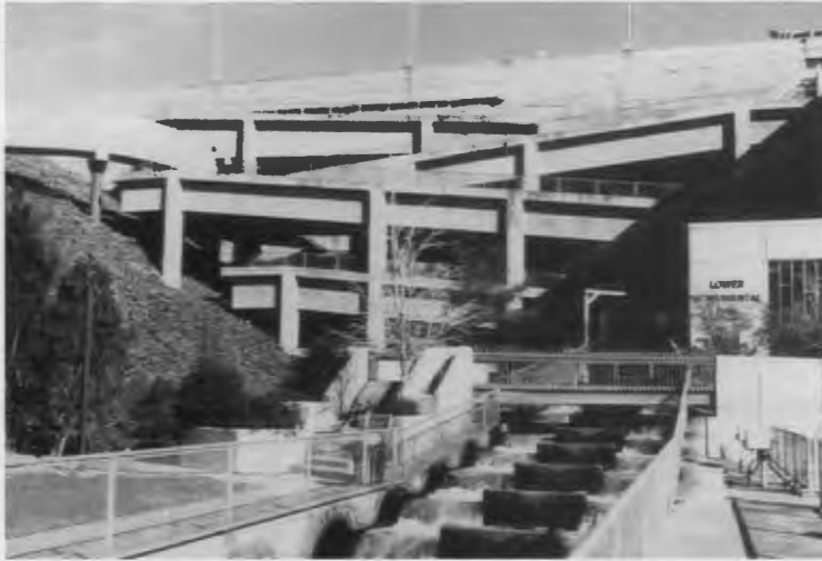
Fish ladder at the Lower Monumental Dam on the Snake River in Washington. This is one of two ladders that allow upstream passage of adult salmon and steelhead above the 100-foot-tall dam. Photograph by Jim Francfort, Idaho National Engineering Laboratory
