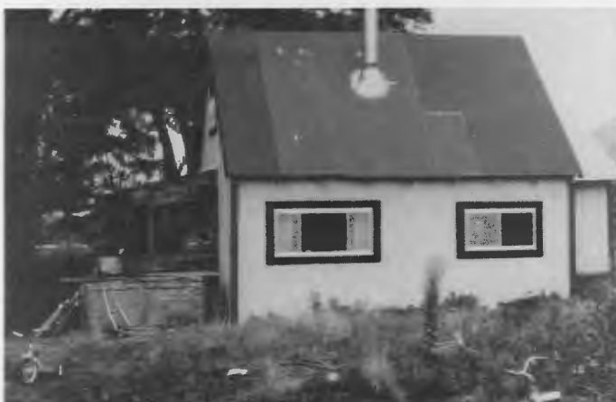
Photographs of a single-family dwelling before and after its energy efficiency was improved by DOE's Weatherization Assistance Program.
