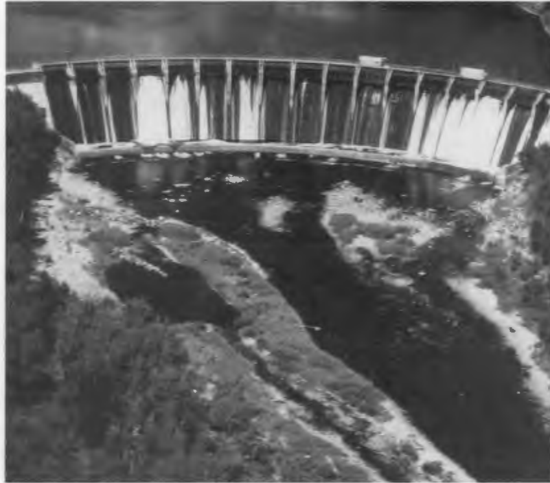
Another view of the Fond du Lac Dam, one of several nonfederal projects being studied by ORNL. Photograph by Mike Sale
