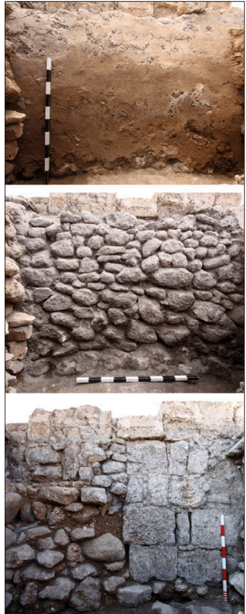
Fig. 3. Mantle against the north wall of building D90: top, clay plaster on the surface; center, stone surface under the plaster; bottom, original wall surface (Photos P. Jaworski)
