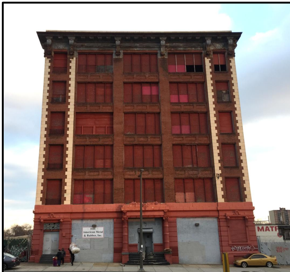
Fig. 5. Above: Looking east at the primary (west) elevation of the subject property. Source: Oscar Beisert, 2018. Source: Pictometry, Atlas, City of Philadelphia, 2018.
