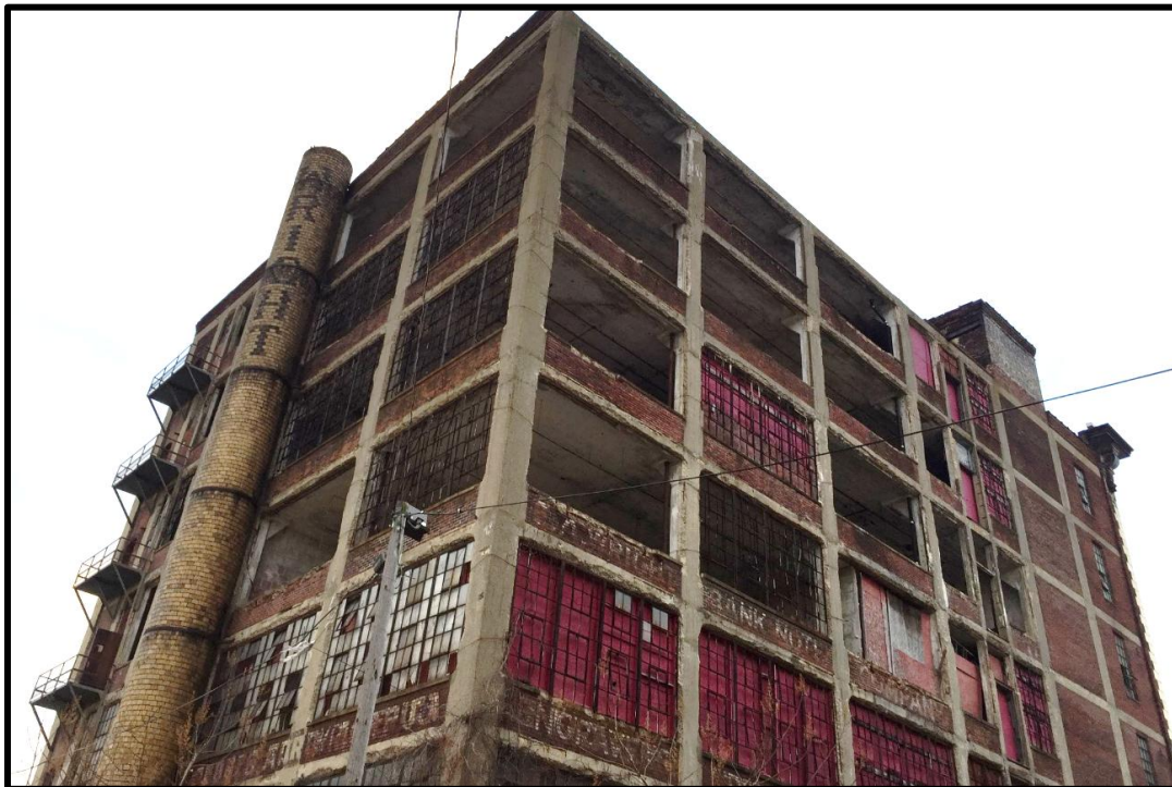
Fig. 14. Looking southwest at the rear (east) and side (north) elevations.
