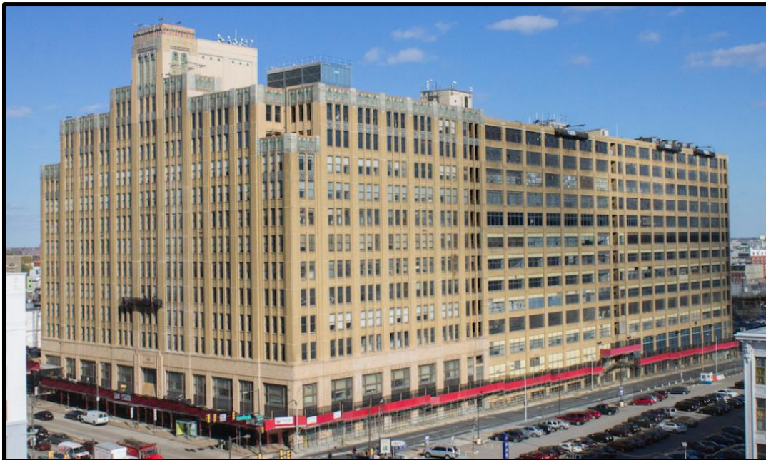
Fig. 40a. Top: The General Electric Switchgear Plant at 421 North 7th Street was built in 1916 by the William Steele & Company for the manufacture of electric switchboards. Source: Wikipedia. Fig. 40b. Bottom: Completed in 1930 by William Steele & Son Company, the Terminal Commerce Building at Broad and Callowhill is of reinforced-concrete construction, being over 30 acres of floor space. Source: Michael Bixler, Hidden City.
