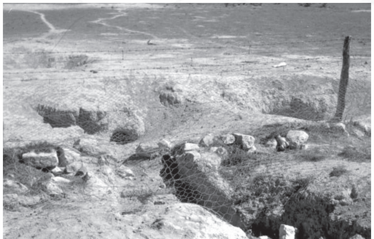
Wombat damage to the Fowlers Bay fence. Courtesy Daryl Rankine. (Photo 102049)
