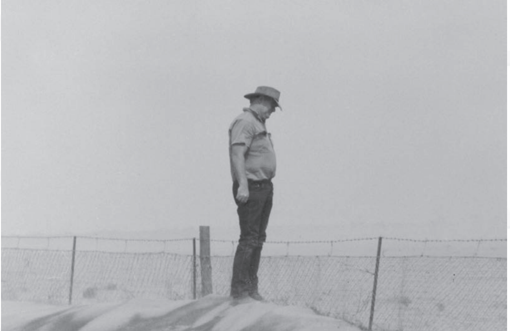
Fence inspector, TV Cook, 1988-97. Old Murat Bay-Petina fence almost covered by sand drift. Courtesy of B A Lock. (Photo 102050)
