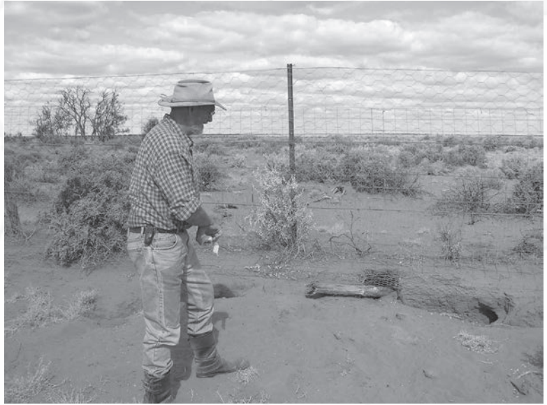
Michael Balharry, during a Fence inspection trip in May 2012, about to attach a piece of tape near a hole in the Fence at Curnamona, so that the patrolman knows to make the necessary repairs. (Photo No.109292)
