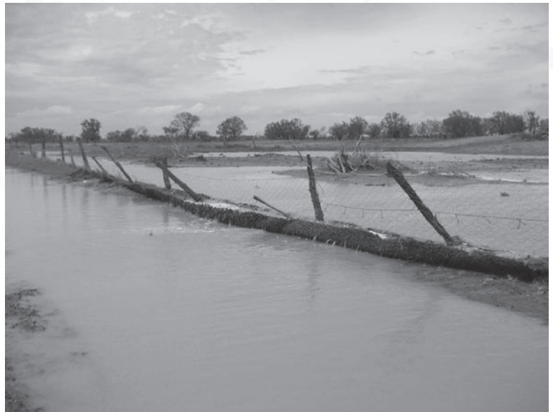
Flood damaged fence at Mulyungarie. (Photo No. 109231)
