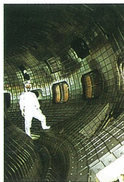
Vacuum Vessel Inside of Vacuum Vessel About ten thousand carbon tiles protect the vacuum vessel from the high temperature plasma. In 1997, the divertor geometry at the bottom of the vacuum vessel was modified, in order to improve the heat and particle flux controllabilities.
