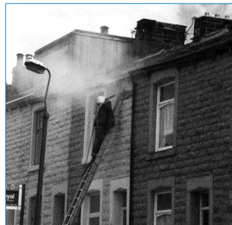
Figure 2.9 Dust generation from sand-blasting (Source: AD Murray, Hynburn BC)
