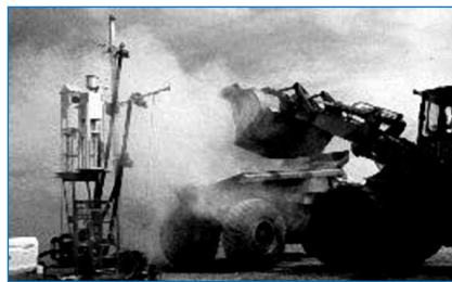
Figure 2.4 Dump truck filling (Source: Midwest Research Institute, USA www.mriresearch.org )
