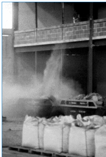
Figure 2.5 Material dropped into skips (Source: BRE Archive)
