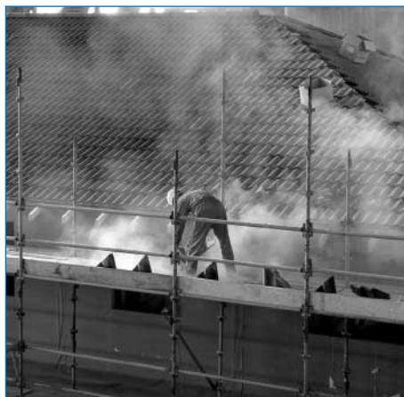
Figure 2.8 Dust generation from disc cutting (Source: BRE Archive)
