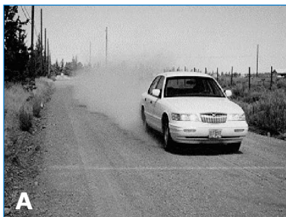
Figure 2.2 Road surface (A) without dust control and (B) with dust control (Source: www.brooksnsw.com.au )
