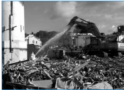
Figure 2.7 Water sprays used to control dust emission during demolition
