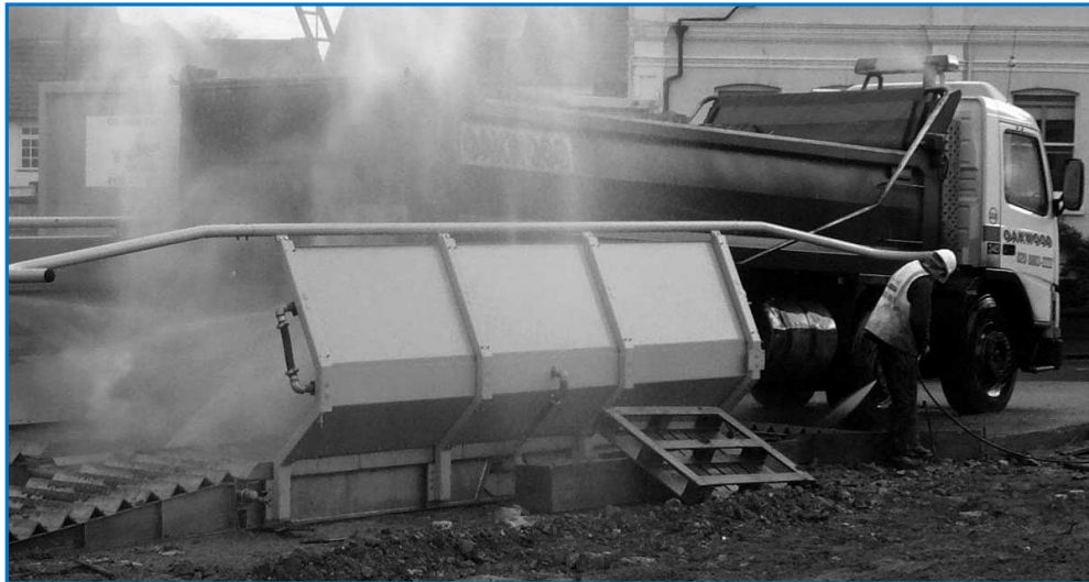
Figure 2.3 Wheel washing of lorry prior to exiting site
