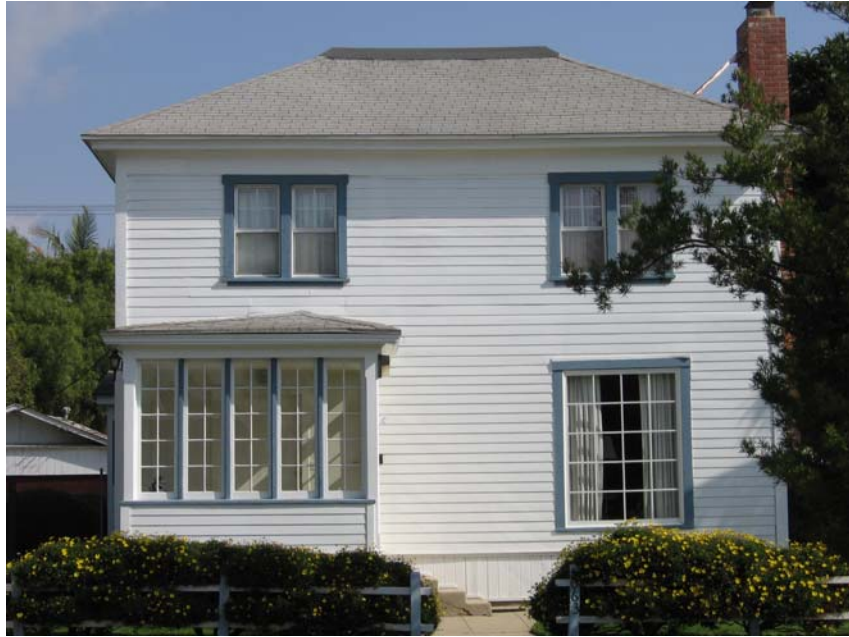
Primary (west) elevation, looking east.
