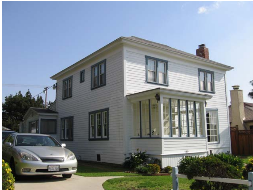
North and west elevations, looking southeast.
