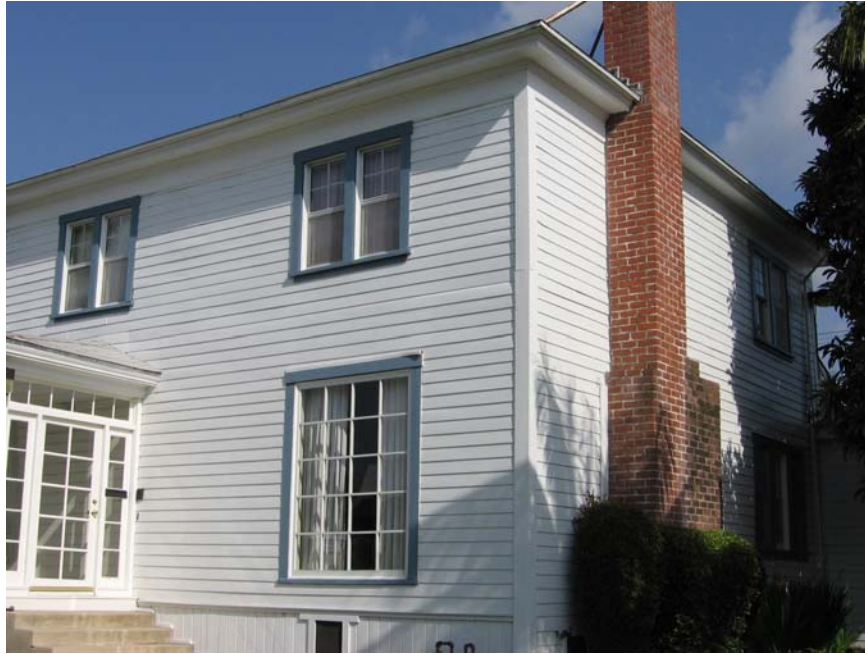
West and south elevations, looking northeast.
