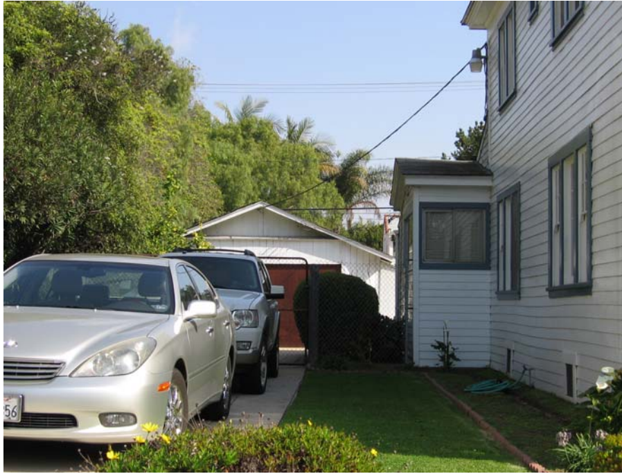
North elevation, secondary entrance. Detached garage. Looking east.
