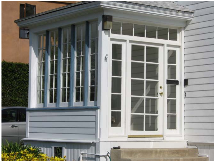
Main entrance, primary (west) elevation, looking northeast.
