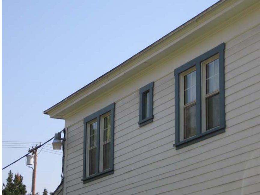
Window detail, north elevation.
