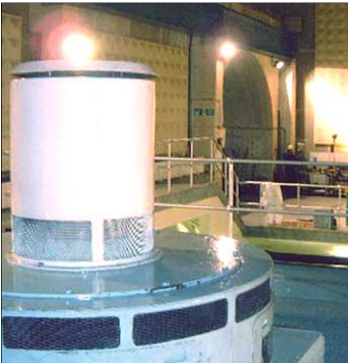
The main generator set at Scottish & Southern's Culligran Power Station by Inverness. Originally 24 MW, its capacity was cut to 17.1 MW prior to the introduction of the Renewables Obligations in April 2002. It is currently being refurbished.
