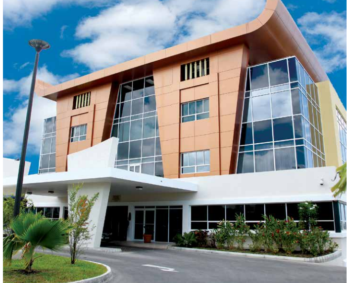
Administration Building – African-influenced
