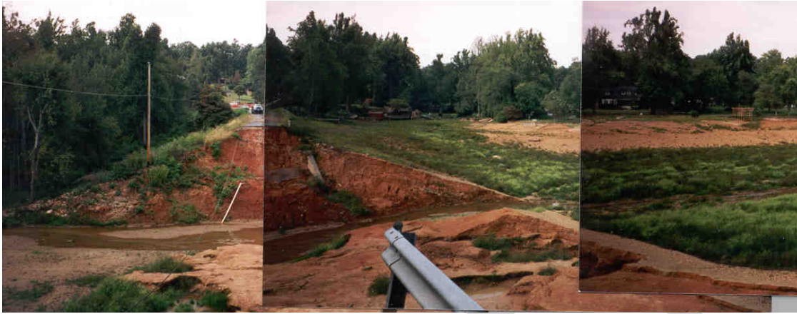
The breached Timberlake Dam Source: Wayne Graham, Reclamation
