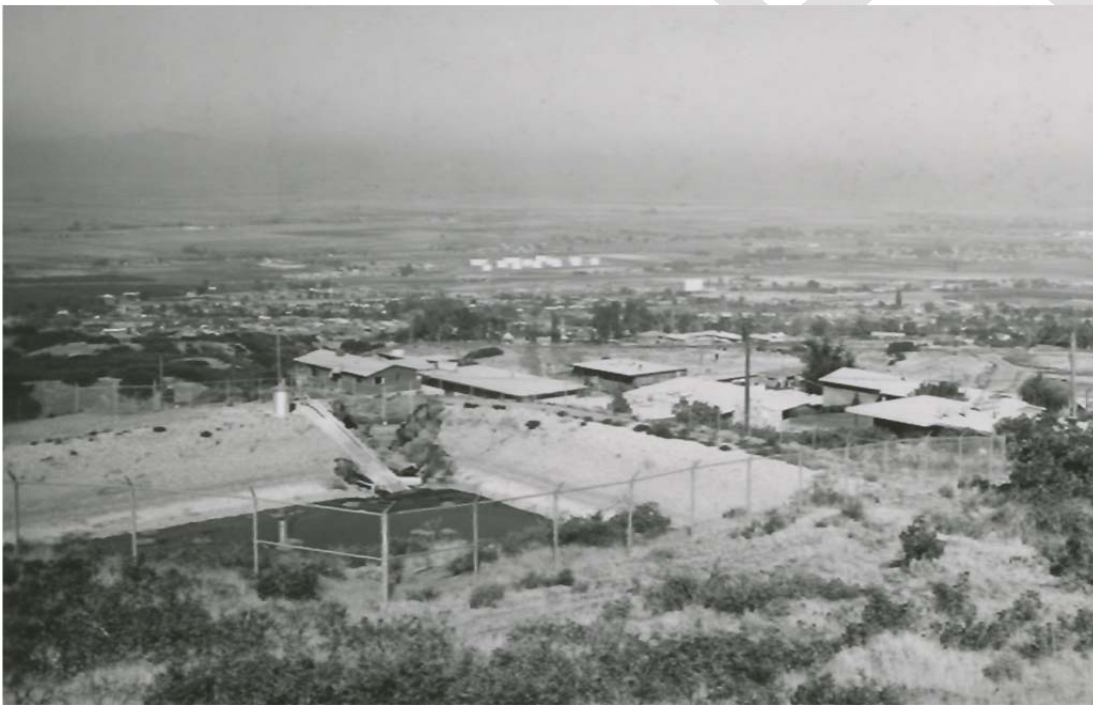
Breached Reservoir No.1 Dam
