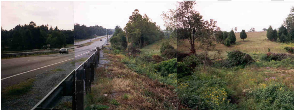
Location where rescue worker was killed Source: Wayne Graham, Reclamation
