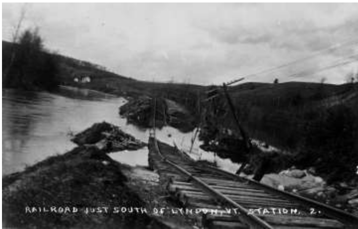
Destroyed railroad tracks Lyndon, VT
