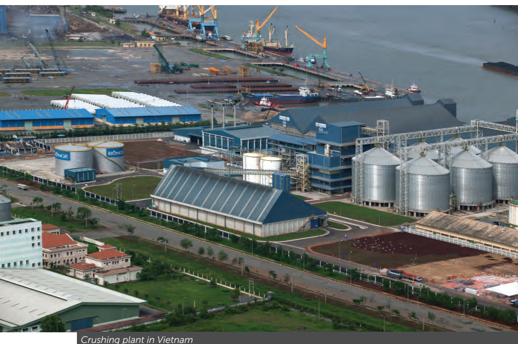
Crushing plant in Vietnam
