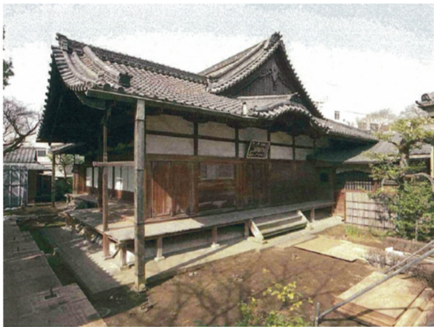
Figure 1: Gekko-den pavilion prior to preservation.
