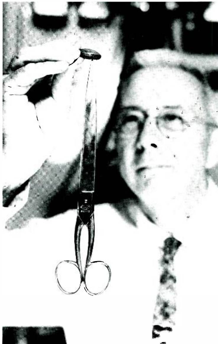
In 1938 E. A. Nesbitt invented a family of permanent magnet materials known as Vicalloys, which are used in the twistor memories of electronic switching systems. Here he demonstrates, in 1968, the strength of one of the most powerful small magnets ever made—"a rare earth" alloy which he helped develop.
