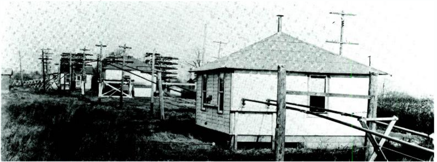
This experimental 1935 installation of large coaxial conductor lines near Phoenixville, Pennsylvania, was the forerunner of
