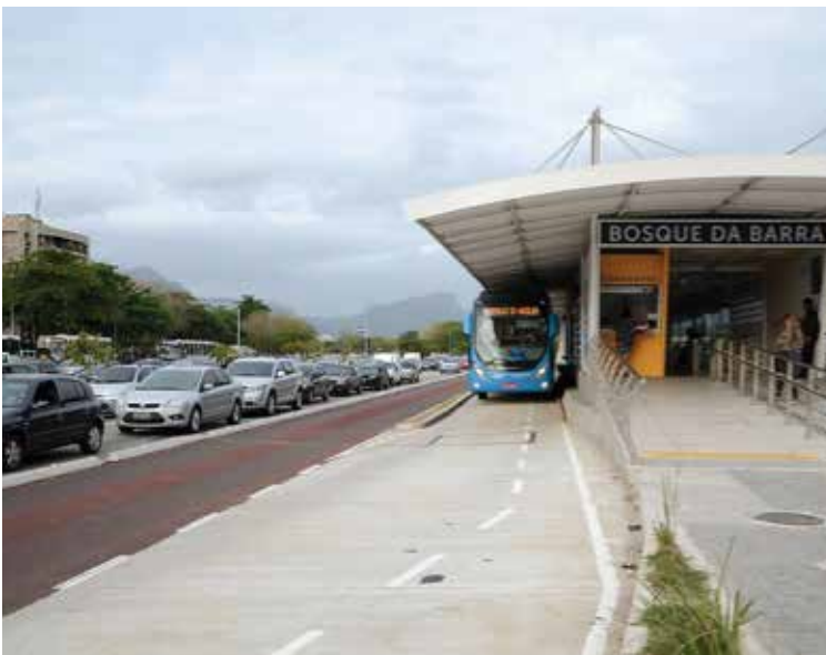
Examples of BRT Systems in Action. Note the dedicated lanes and above-grade, high-quality stations with level passenger boarding.
