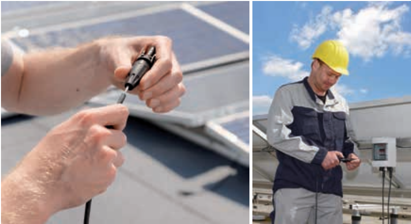
Figure 62 and 63: Push-in connector for field assembly on a PV module Figure left: source: Weidmüller, Figure right: source: Phoenix Contact
