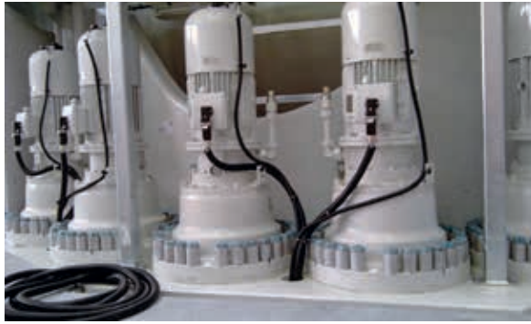
Figure 60: Connectors connecting motors which align the turbine rotor blades with the wind direction (yaw) – source: Harting
