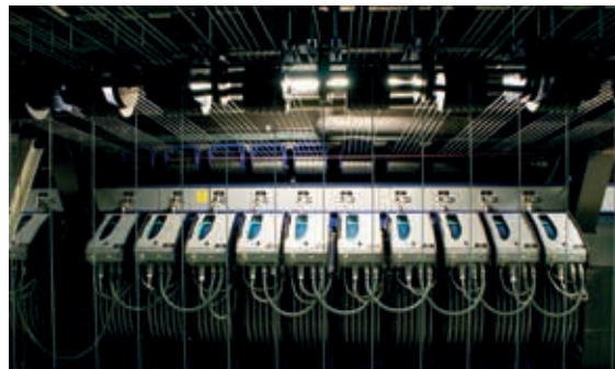
Figure 73: Cable winch control system for a musical at the London Palladium Theatre – source: Courtesy of Trekwerk
