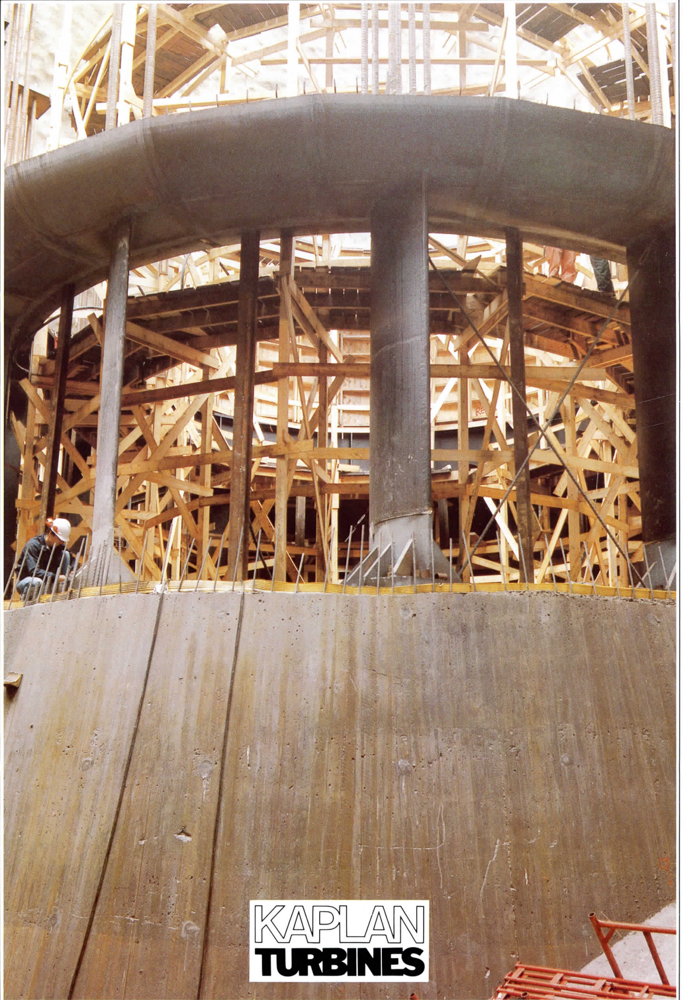
Solbergfoss staying under assembly
